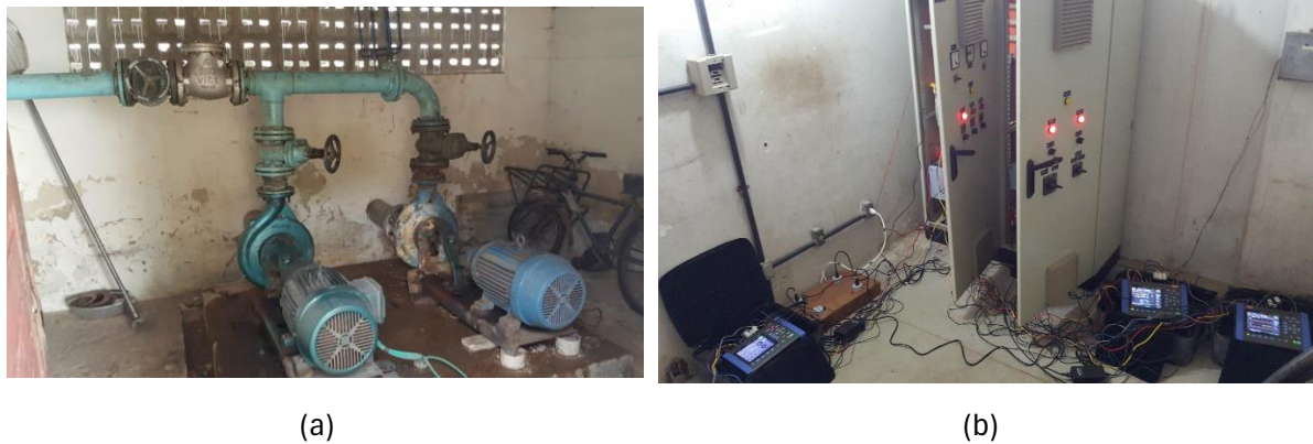
Figure 7-9 – Pumping System at the Federal University of Pará: (a) 15 kW SCIM and (b) Power quality analyzer for electric motors consumption measurement.
